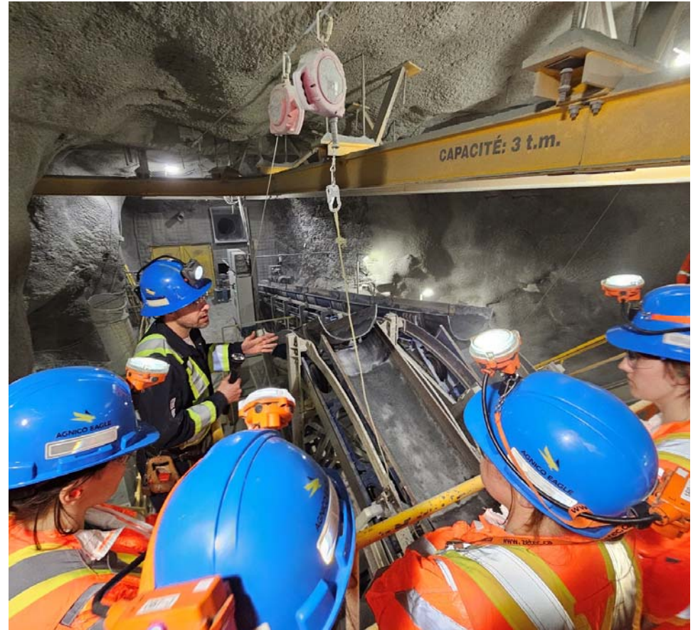
Taking a look at the railveyor system
